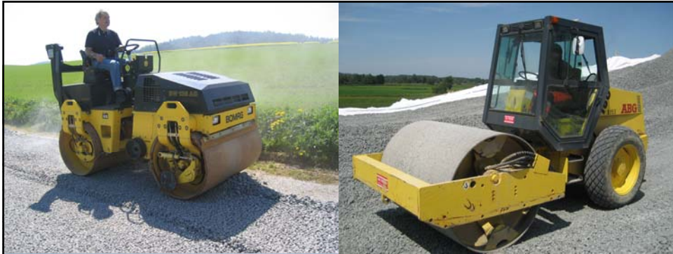
Dynamic roller compaction
