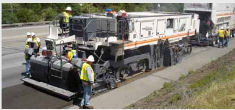
Recycling of the right shoulder with the WR 4200
