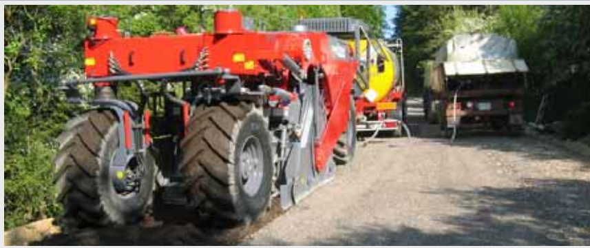
Recycling of tarry asphalt granulate by adding bitumen emulsion and water
