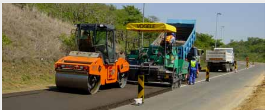
Paving 125 mm thick layer with Vögele Paver
