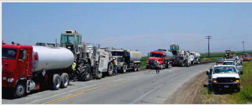
Highway 20 recycling with foamed bitumen
