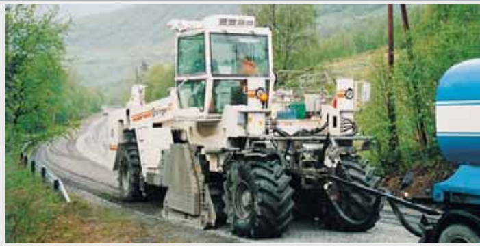
Cold Recycling with bitumen emulsion; (pre-spread aggregate)
