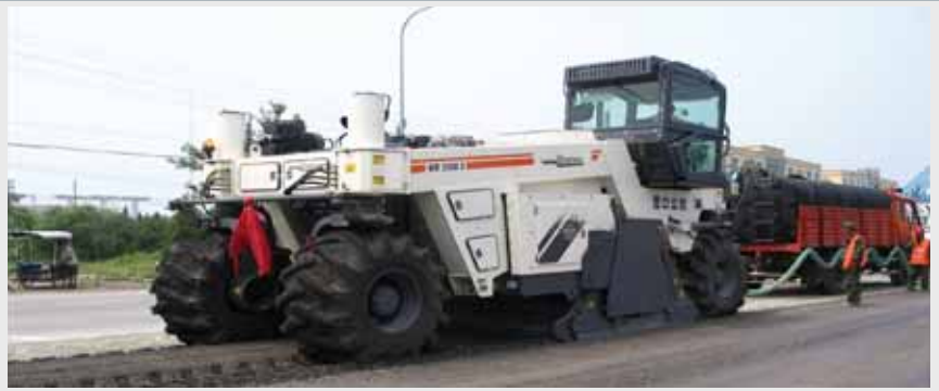
Cold in place recycling with bitumen emulsion and cement Yingkou/Liaoning Province
