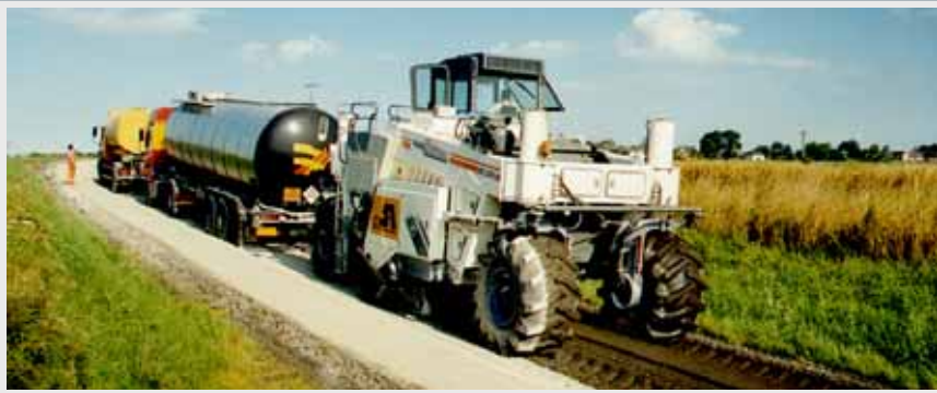
Cold Recycling with bitumen emulsion and cement with the WR 2500 S
