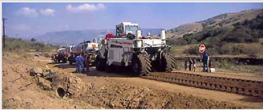
Upgrading an unbound gravel road by Cold Recycling with foamed bitumen
