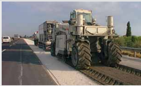
In situ Cold Recycling with cement slurry and foamed bitumen
