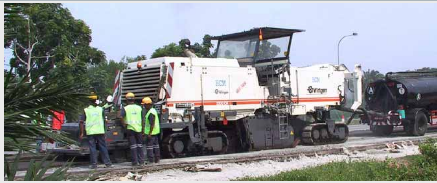
Recycling with cement + emulsion
