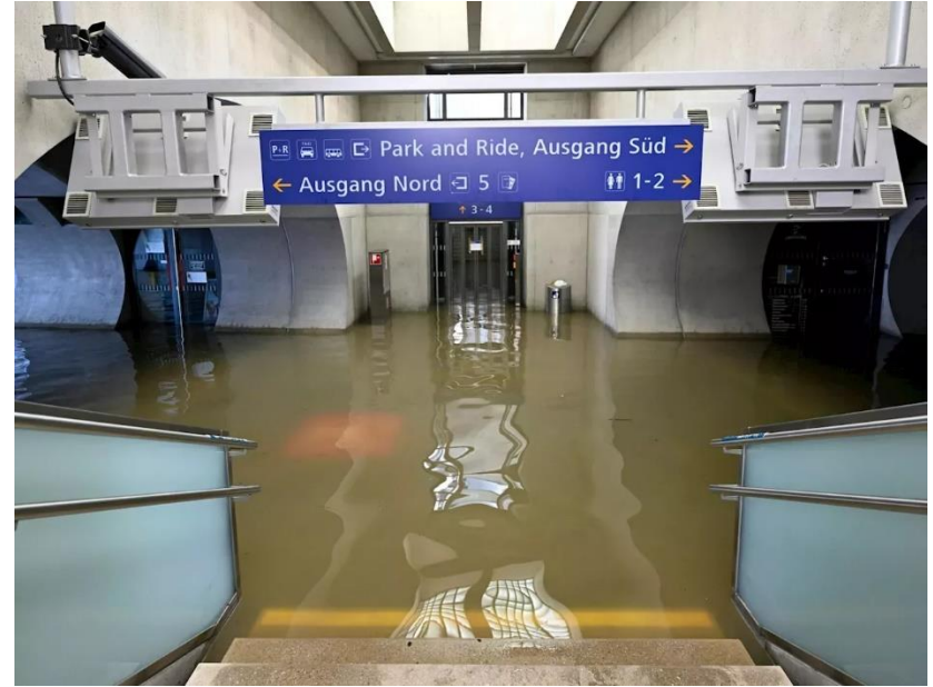
flooding in Eastern Austria, station Tullnerfeld, Sep 2024 (ÖBB)
