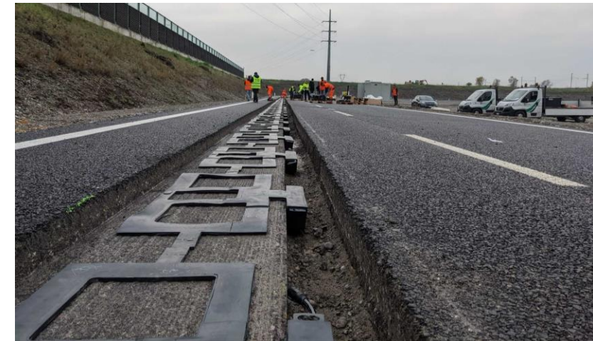
Electreon: in-road inductive
