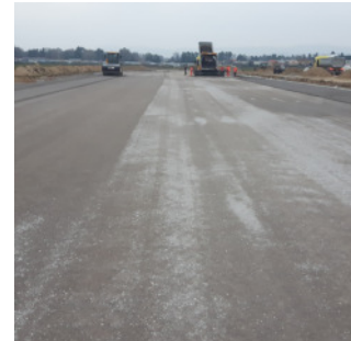
Verification in the practice
