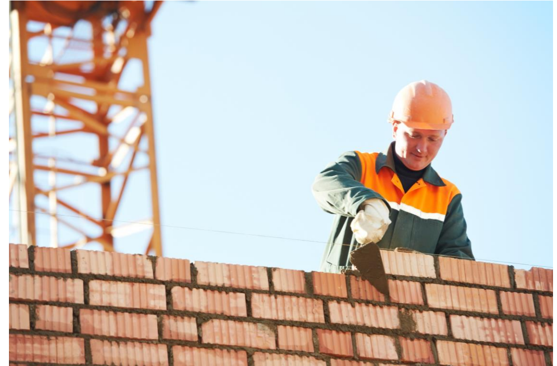
Brickwork construction today
