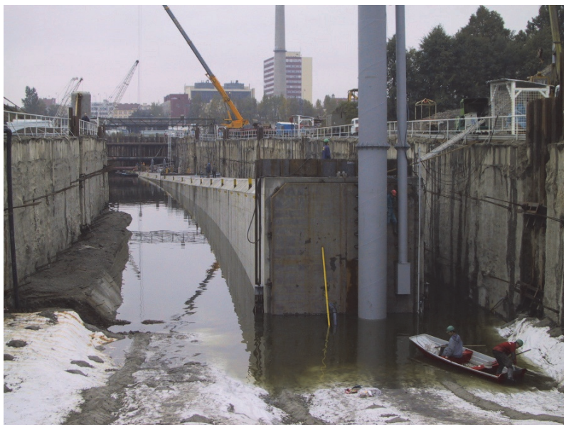
Fig. 15. A partially flooded dry dock with the tunnel tube
