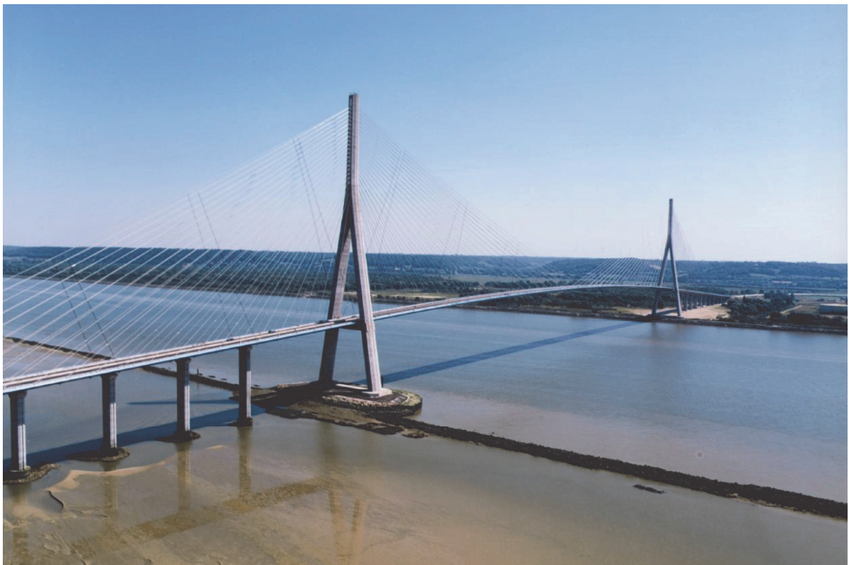
Fig. 19. The Normandie Bridge
