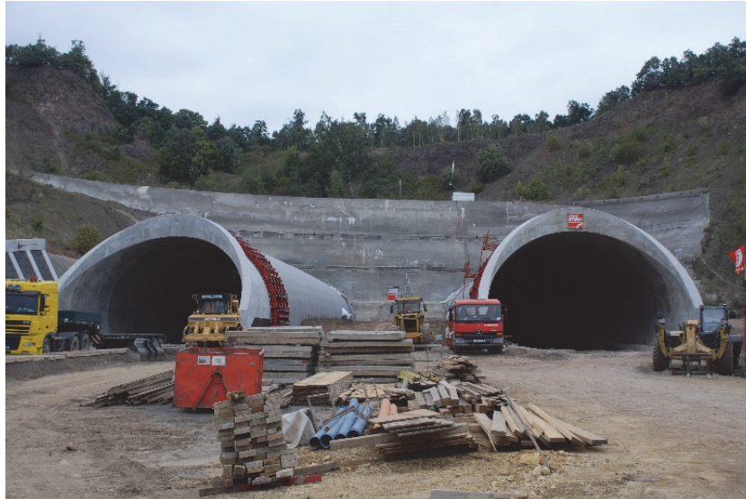
Fig. 3. Portal of the Prackovicky tunnel – motorway D8 Prague - Dresden
