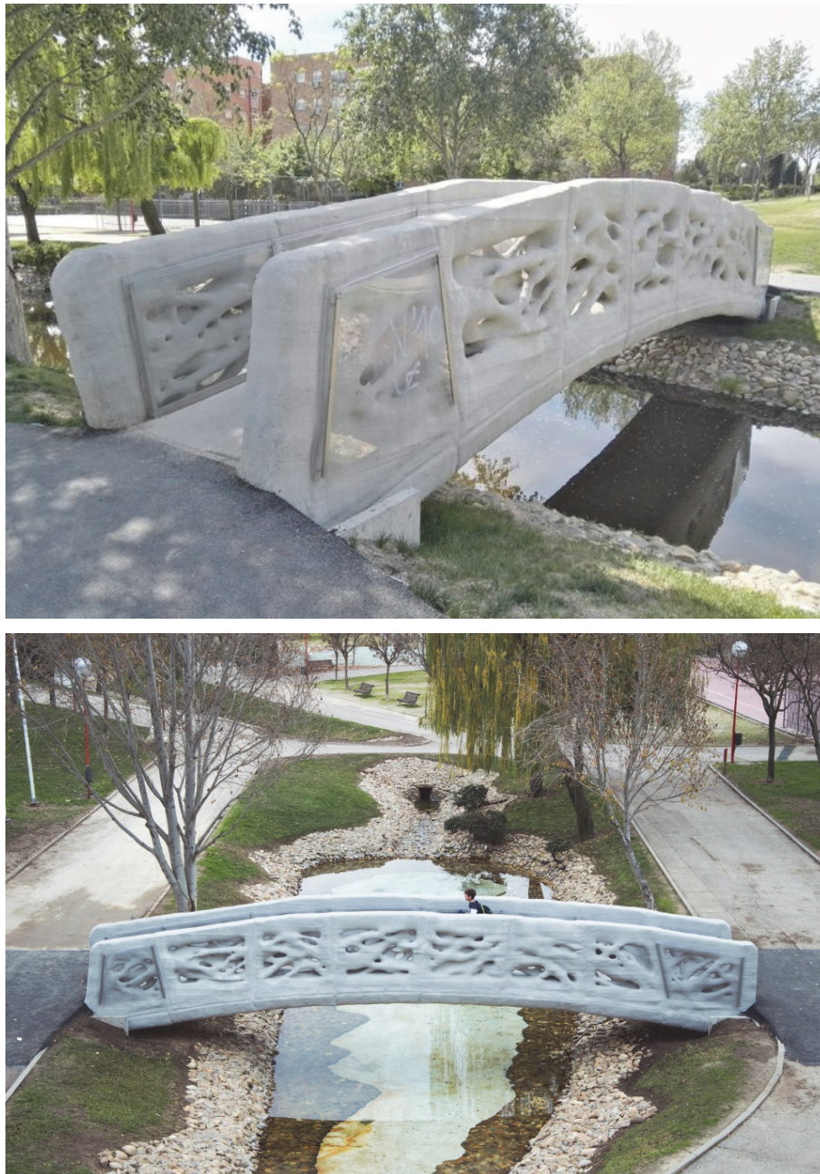
Fig. 4. 3D concrete printed pedestrian bridge in Alcobendas (Madrid, Spain) completed in 2016 (De la Fuente, Blanco, Galeote, Cavalaro, 2022)
