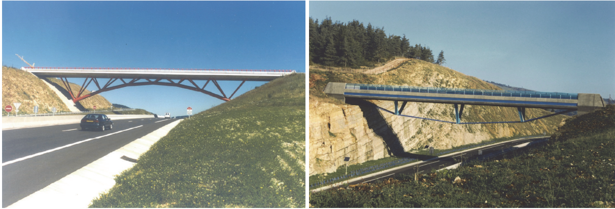
Fig. 8. The Antrenas Bridge (left) and the Truc de la Fare Bridge (right)
