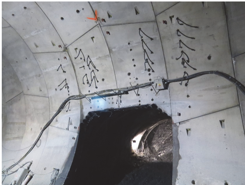
Fig. 10. Opening in the precast lining for the connecting gallery
