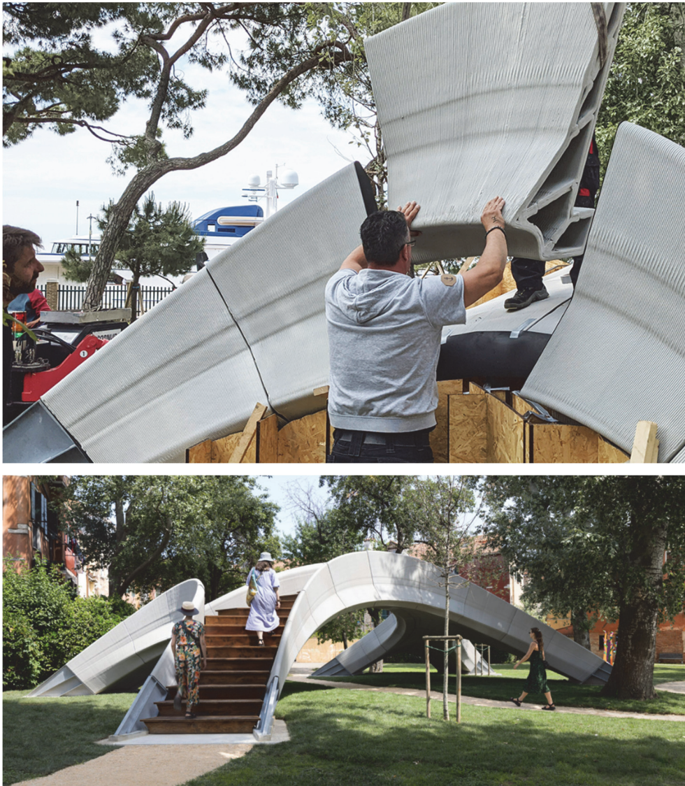
Fig. 5. 3D concrete printed pedestrian bridge (Venice Biennale, Italy) concrete blocks without reinforcement completed in 2021 (ETH Zurich, BRG, Architects, Z.H., CODE, Incremental3d, HOLCIM, 2022)
