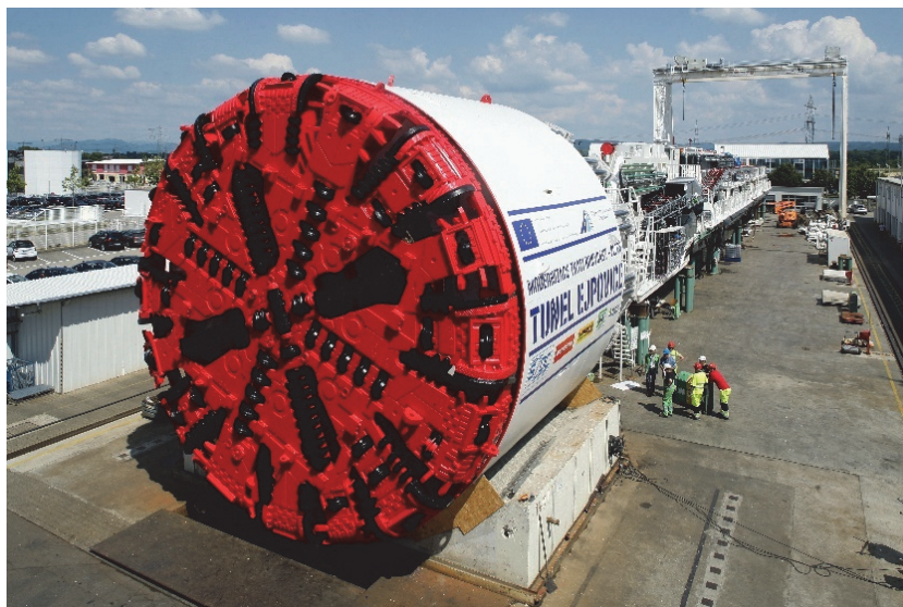
Fig. 8. TBM used for the construction of the Ejpvovice railway tunnel
