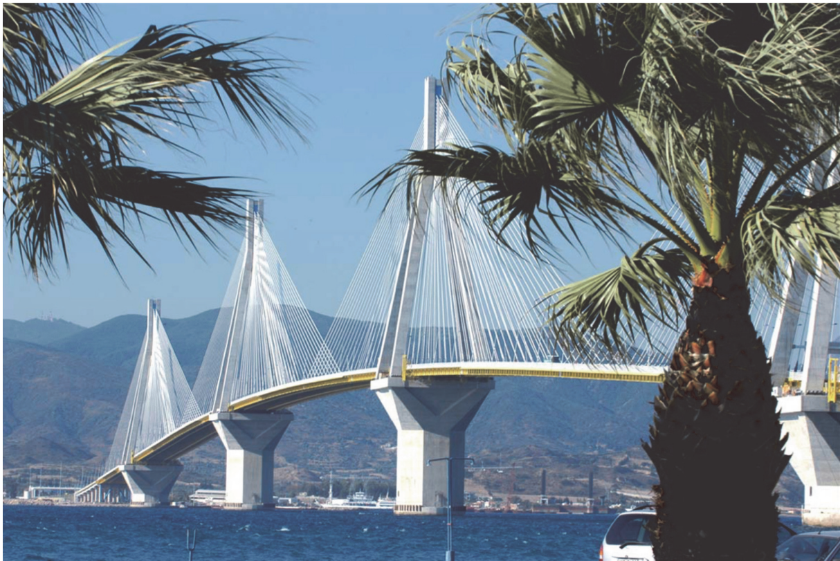
Fig. 17. The Rion-Antirion Bridge
