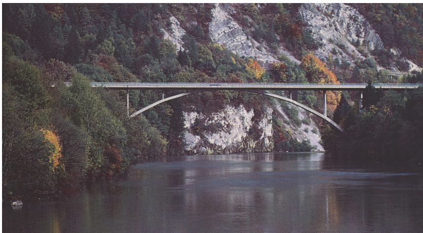
Fig. 4. A bridge on the River Rhein (Christian Menn)
