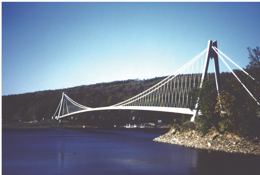
Fig. 7. The Swiss Lake Bridge Czech Republic (Jiri Strasky)
