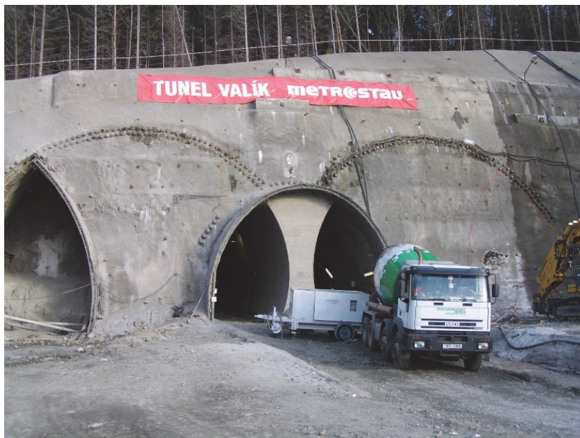
Fig. 4. Central pillar of the Valik tunnel before excavation of main tunnels
