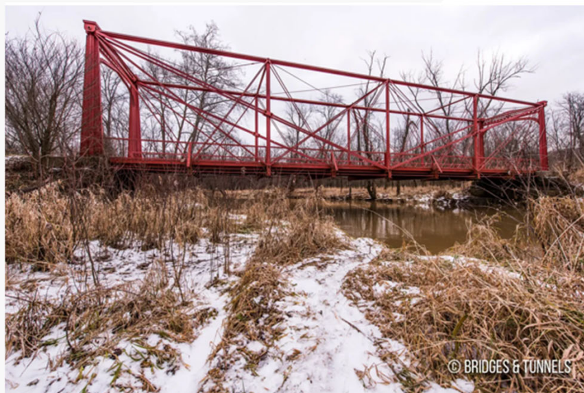
Zoarville Station Bridge
