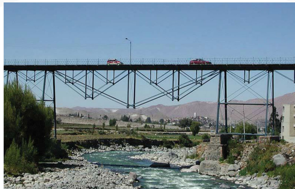
Rio Chili Bridge
